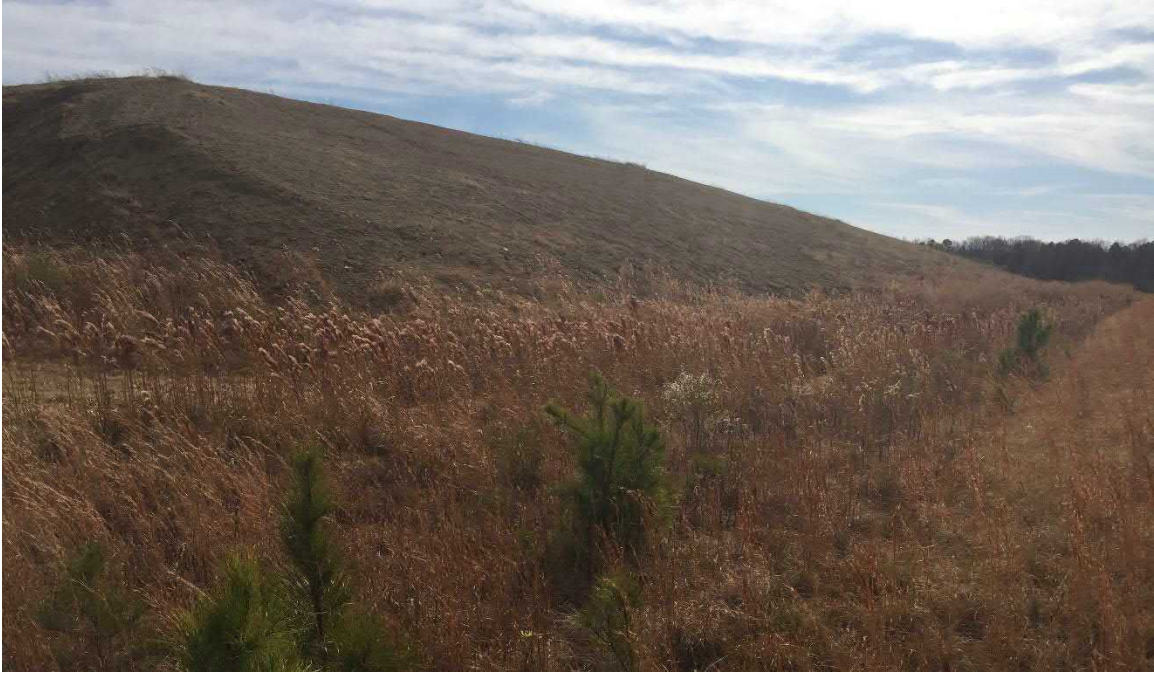
7. Looking south across west slope of Cell 3
