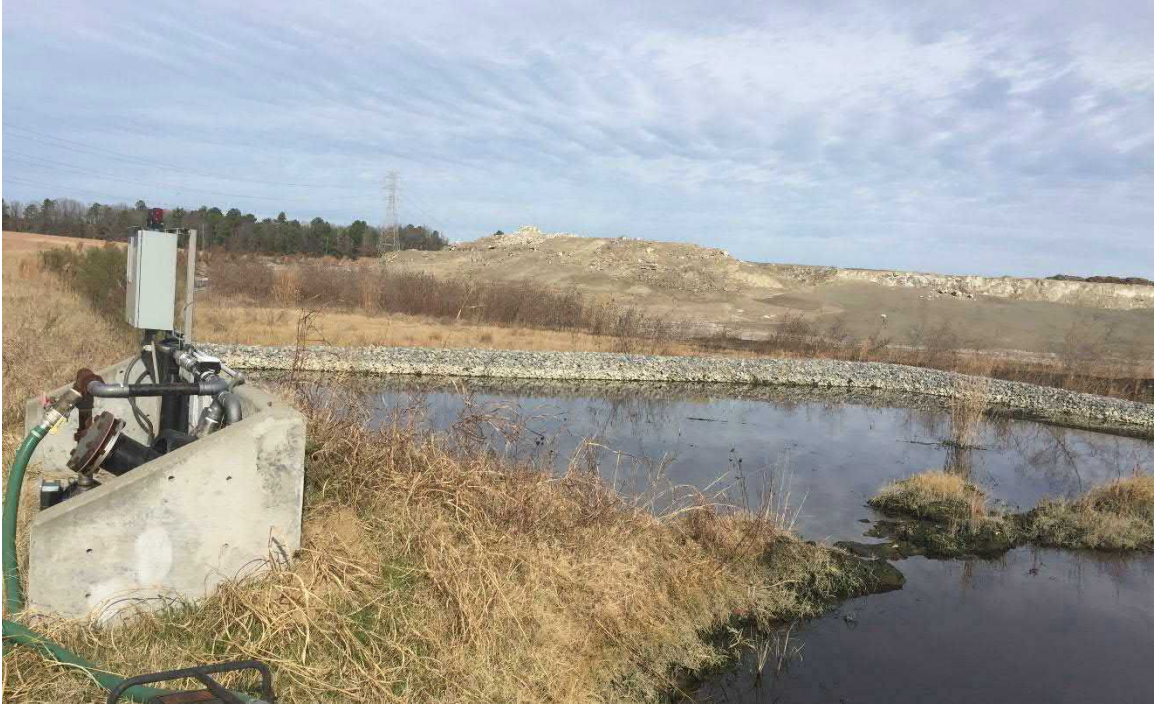
3. Looking north at Cell 4 sump.
