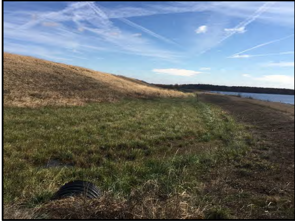
7. South side of Phase 1 looking east.
