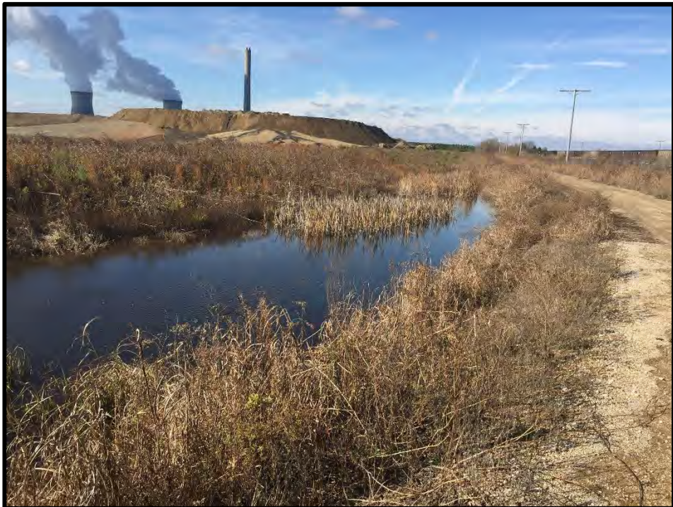
4. Cell 1 east dike looking to the south. This slope drains to the east and into the storm water runoff pond.
