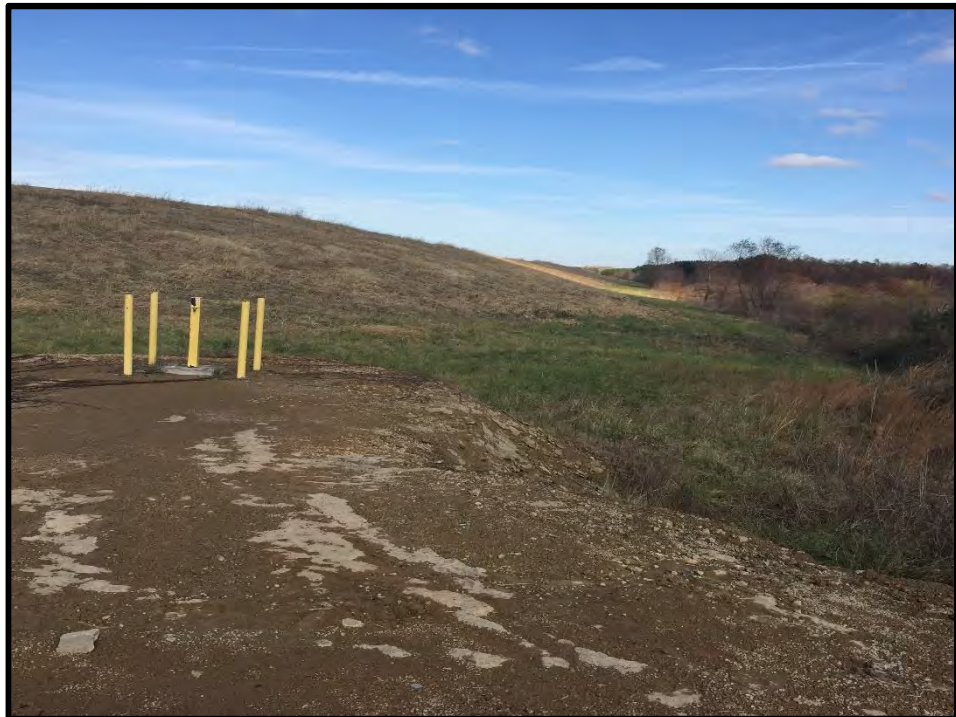
8. East of Phase 1 looking north.
