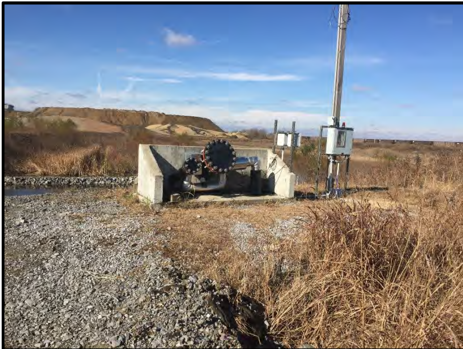
2. Cell 1 north dike looking to the west. The ash is kept away from the north dike to assist with leachate management.
