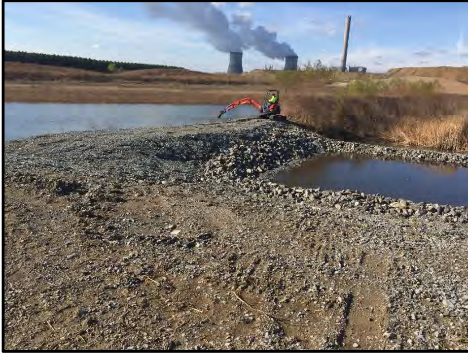
1. Cell 15 sump area. Headwaters is performing general maintenance by the Cell 15 Sump.
