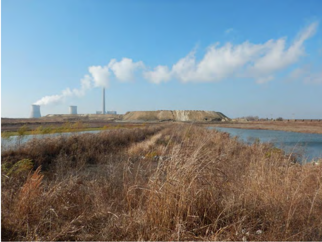
Photo 3. Leachate sump in Cell 15 looking west.
