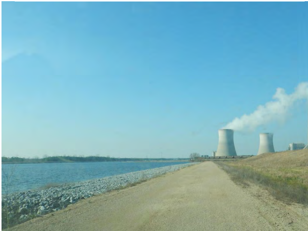
Photo 4. Landfill perimeter access road looking west.
