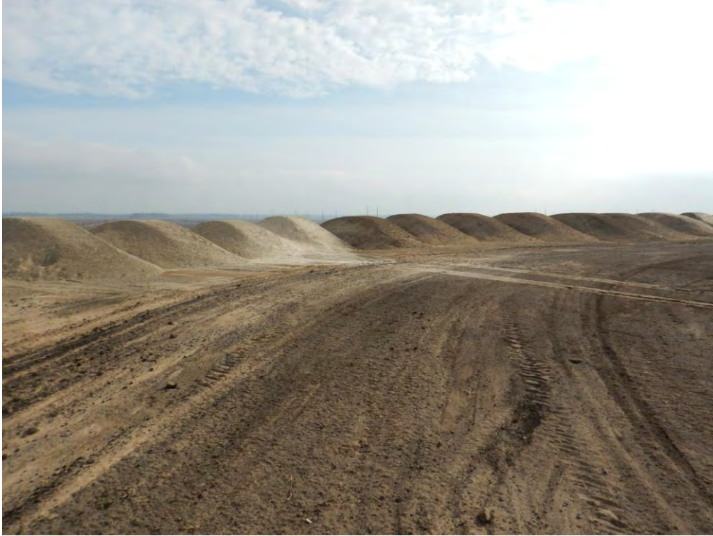
Photo 1. Active working face in Cell 15 looking southeast.
